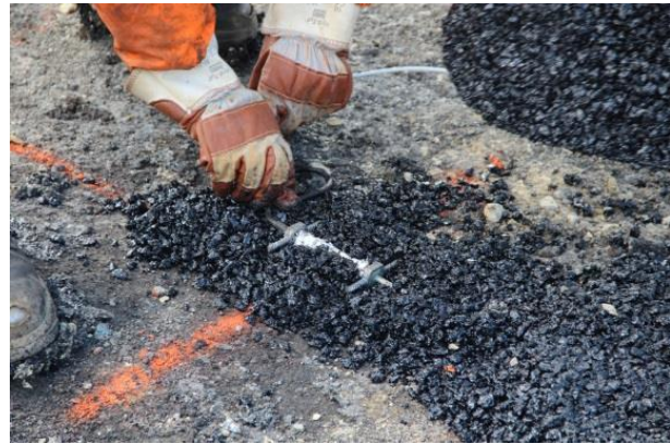
b) Installation of strain gauges prior to paving operation
