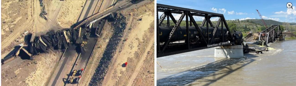
Figure 1. Two significant derailment failures: Left: 30 BNSF rail cars hauling coal near Pueblo, Colorado, derailed on October 15, 2023, causing extensive damage and one death on I-25 below the bridge (photo courtesy of KVDR); right: 16 rail cars, 15 of which had hazardous material, derailed on June 24, 2023 at Reed Point, Stillwater County, Montana (photo NTSB). In the former case, the tracks had been inspected on the day of the accident.
