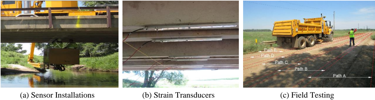
Figure 1. Bridge Field Testing (Rimal et al., 2021)
