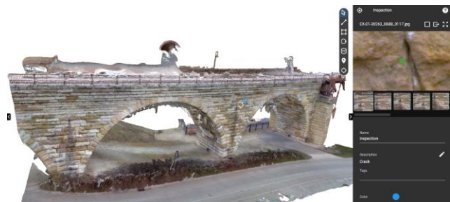
(b) 3D Reconstructed Bridge (Wells and Lovelace, 2018)
